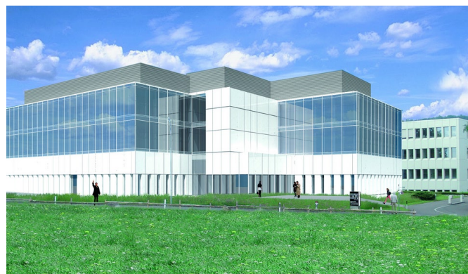
The newly built four-floor Binnig and Rohrer Nanotechnology Center boasts over 950m 2 of clean rooms and 176m 2 of noise-free labs.
